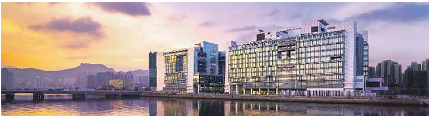
Kembla® Medical Gas Copper Tube has been installed on some of the largest projects in the world over the last 60 years. (Hong Kong Children's Hospital pictured).
