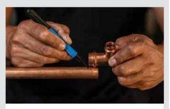
4. Mark the insertion depth by lining up the fitting side by side with the tube and mark the tube. When the fitting is inserted onto the tube the outer edge of the fitting must line up with the marking. For correct insertion depths see column **E** of the Fittings Space Requirements table, page 29.
