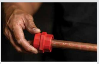
2. Deburr carefully the end of the tube on the inside to minimise turbulence and pressure loss according to AS3500 and on the outside to avoid damaging the O-ring.
