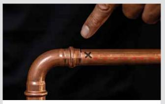
**9.** Visually inspect the fitting to ensure the press has been completed. The KemPress® tool will flash if the fitting did not press correctly. If this occurs a new fitting and tube section is required. At the end of the project visually inspect each fitting to ensure none have been missed. By simply marking each press on your KemPress NZ fitting with a marker or spray you can easily identify unpressed fittings and audit installations visually with the naked eye.
