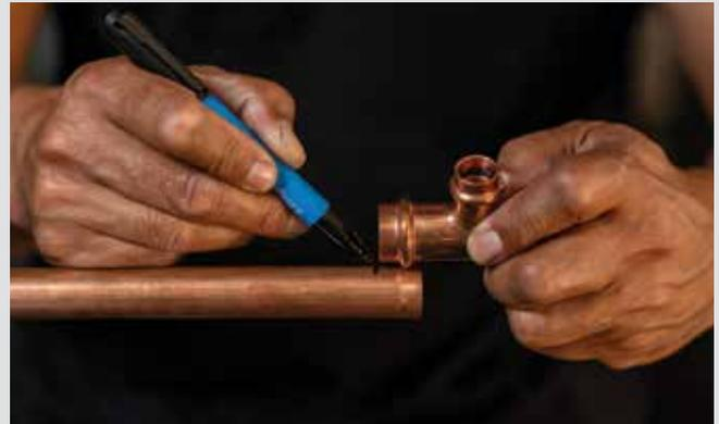
**4.** Mark the insertion depth by lining up the fitting side by side with the tube and mark the tube. When the fitting is inserted onto the tube the outer edge of the fitting must line up with the marking. For correct insertion depths see column **E** of the Fittings Space Requirements table, page 29.
