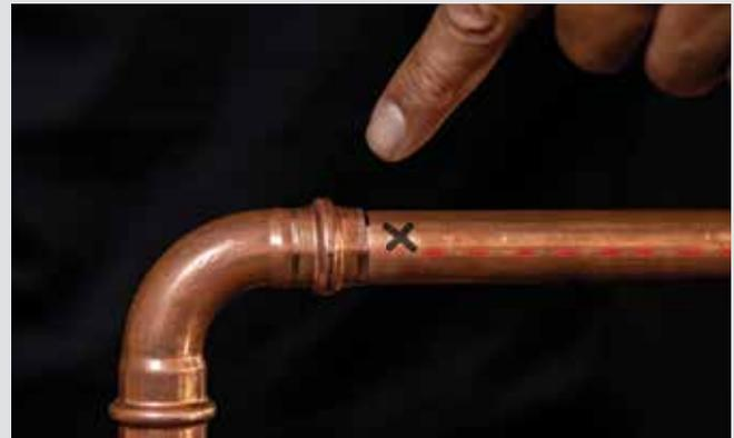
**9.** Visually inspect the fitting to ensure the press has been completed. The KemPress® tool will flash if the fitting did not press correctly. If this occurs a new fitting and tube section is required. At the end of the project visually inspect each fitting to ensure none have been missed. By simply marking each press on your KemPress NZ fitting with a marker or spray you can easily identify unpressed fittings and audit installations visually with the naked eye.
