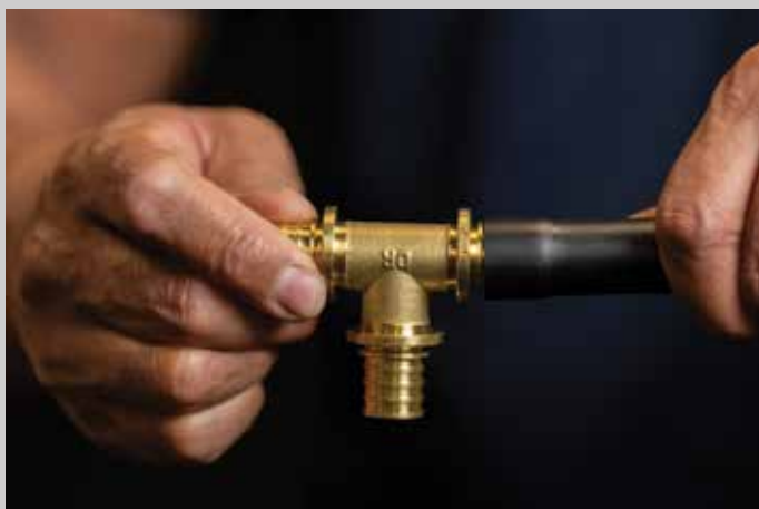
7. Ensure fitting is inserted into shoulder stop and all fitting ribs are covered by the pipe.
