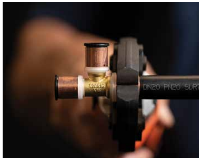
4. Position KemPex crimping tool over the copper sleeve making sure they are square and alongside the shoulder.
