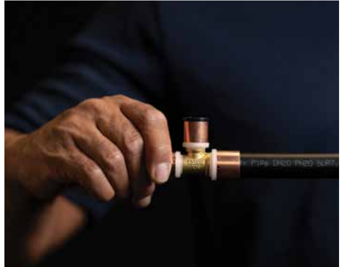
2. Fully insert KemPex Crimp fitting.
