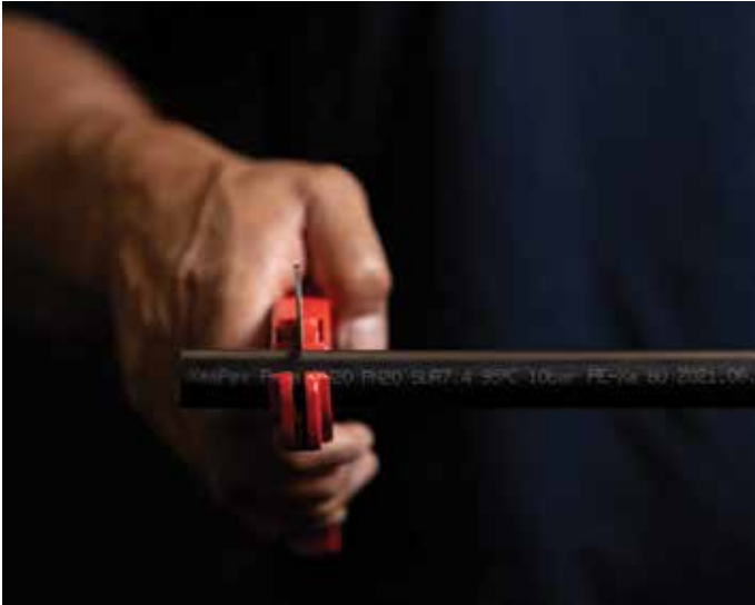
1. Cut KemPex pipe at right angle ensuring you have a straight neat cut to start
